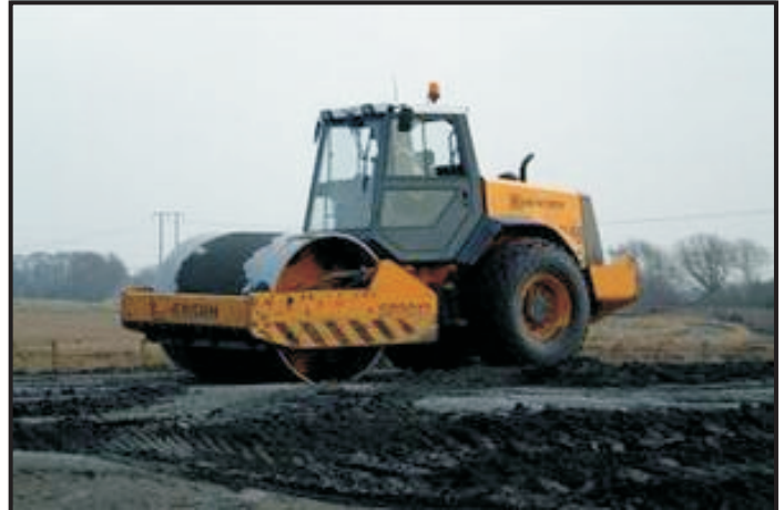
Truck paving road with coal ash
