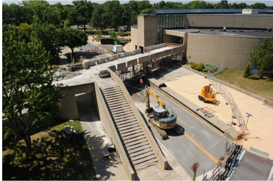
Spine bridge demolition.
