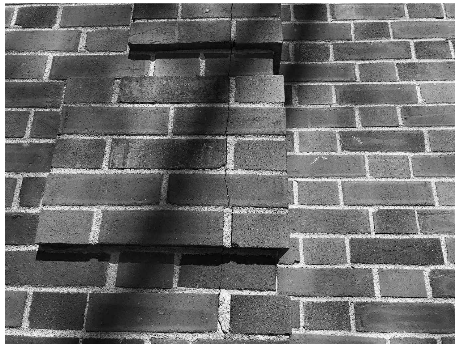
3 PHOTO - TYPICAL BRICK DAMAGE @ CORNER SCALE: N/A
