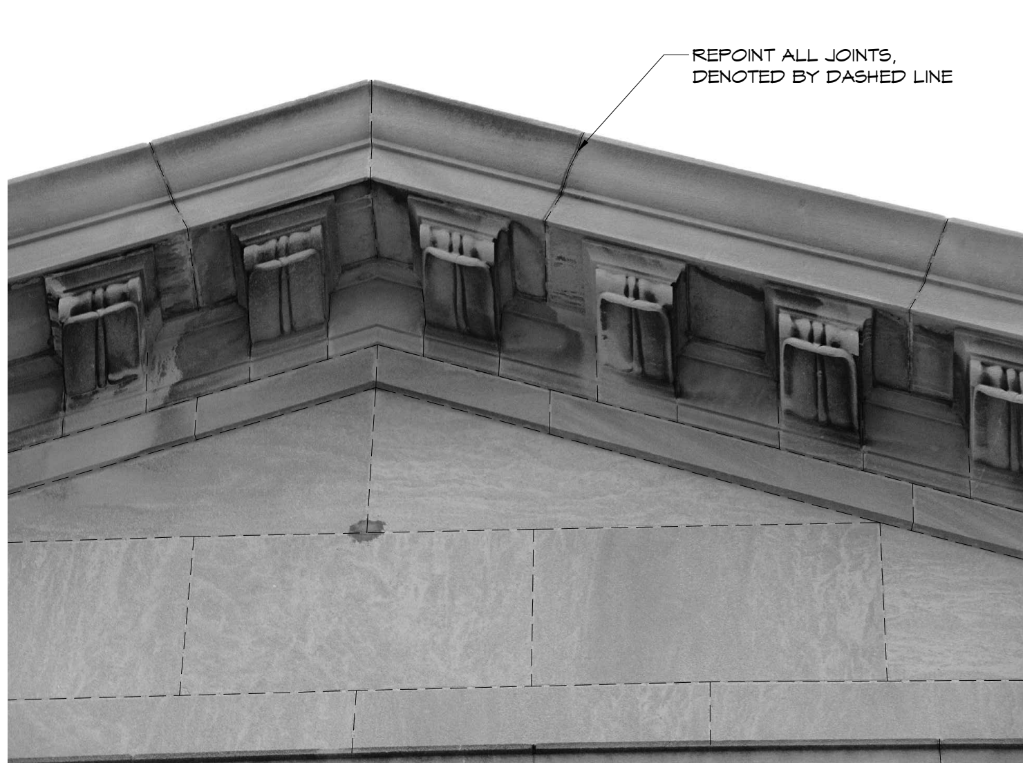
6 PHOTO - LIMESTONE DETAIL AT PEDIMENT 01 SCALE: N/A
