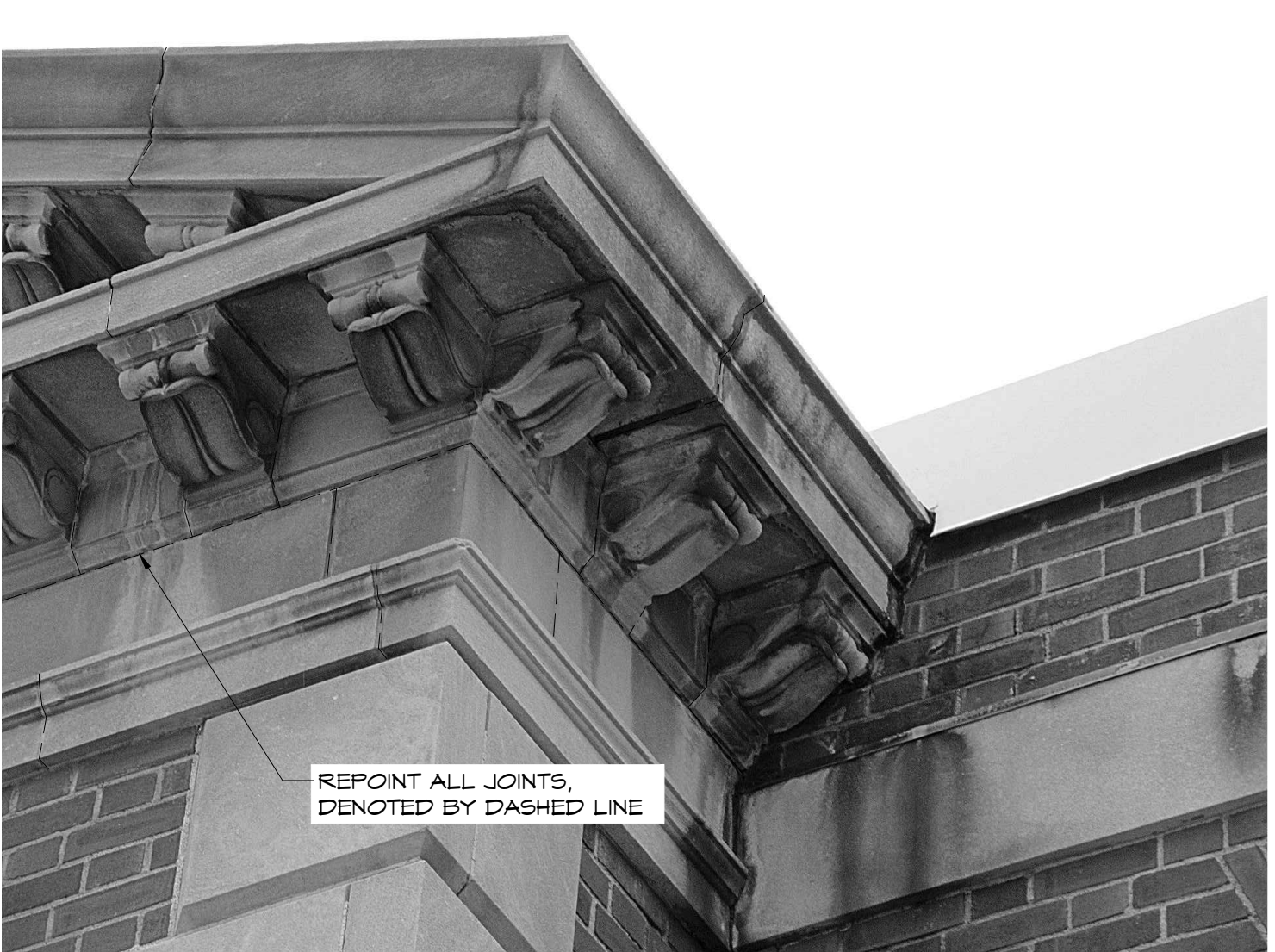
8 PHOTO - LIMESTONE DETAIL AT PEDIMENT 03 SCALE: N/A
