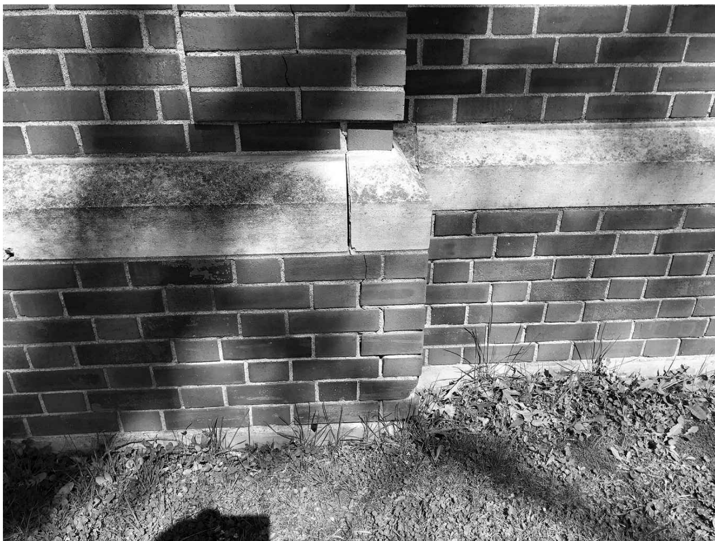
4 PHOTO - TYP. WATER TABLE STONE @ CORNER SCALE: N/A
