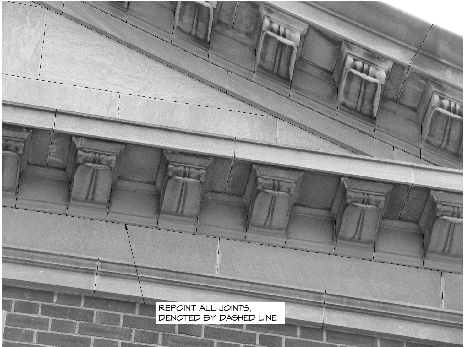
7 PHOTO - LIMESTONE DETAIL AT PEDIMENT 02 SCALE: N/A
