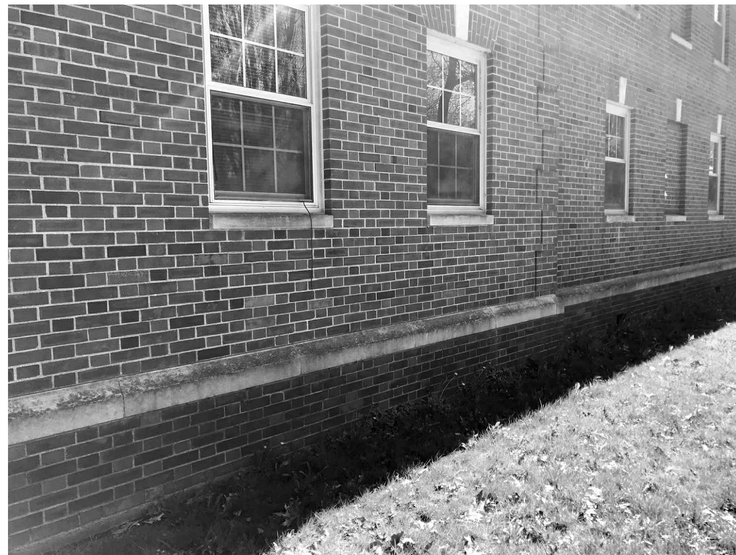
5 PHOTO - TYPICAL WATER TABLE STONE SCALE: N/A
